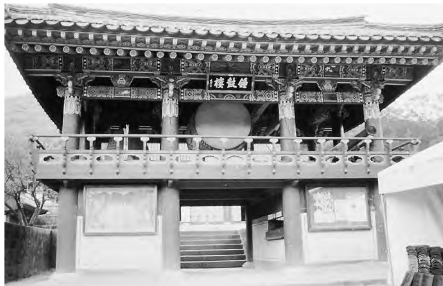
Drum and Bell Tower
